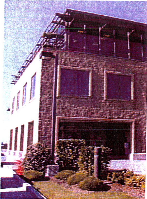
In this case, third story articulation breaks up the perceived bulk of the building
