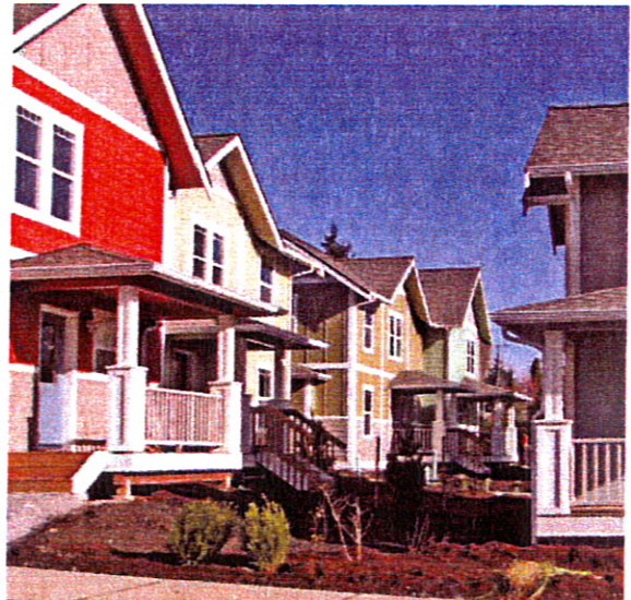
Roof pitches, dormers and change in upper level materials break down the scale of a multi-family development and relate to single family character nearby
