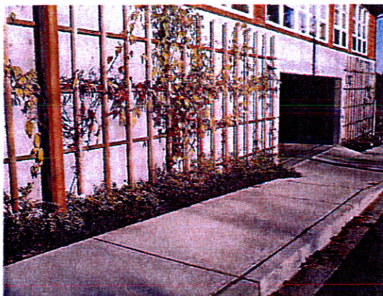
Ground cover and vines help soften a flat facade
