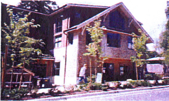
Vary the three dimensional character of the building from bottom to top
