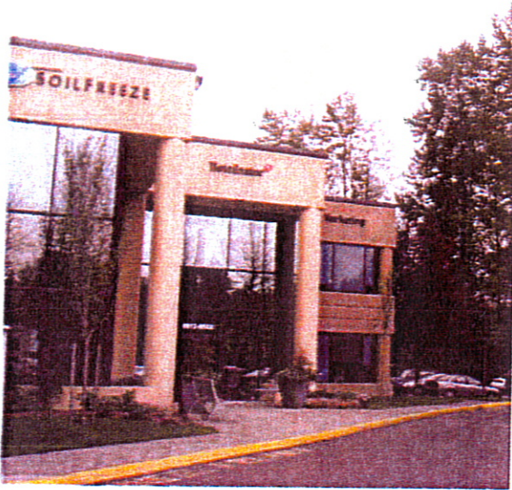
Double height glazing, columns and landscaping give prominence and identity to a main building entrance
